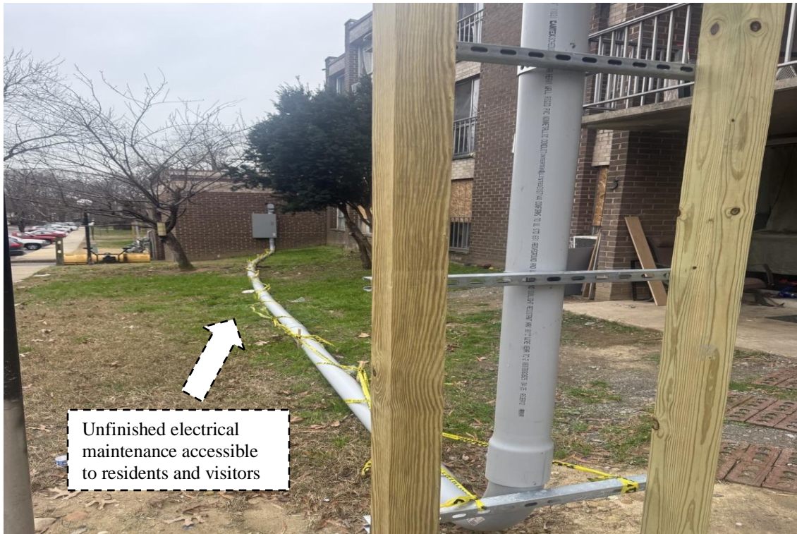
7967 Riggs Rd, accessible unfinished Electrical maintenance
