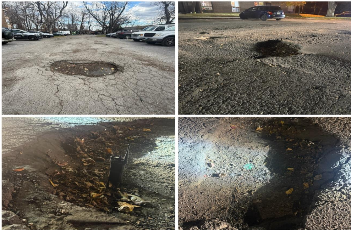
Large potholes in the parking lot between 7975-7979 Riggs Rd
