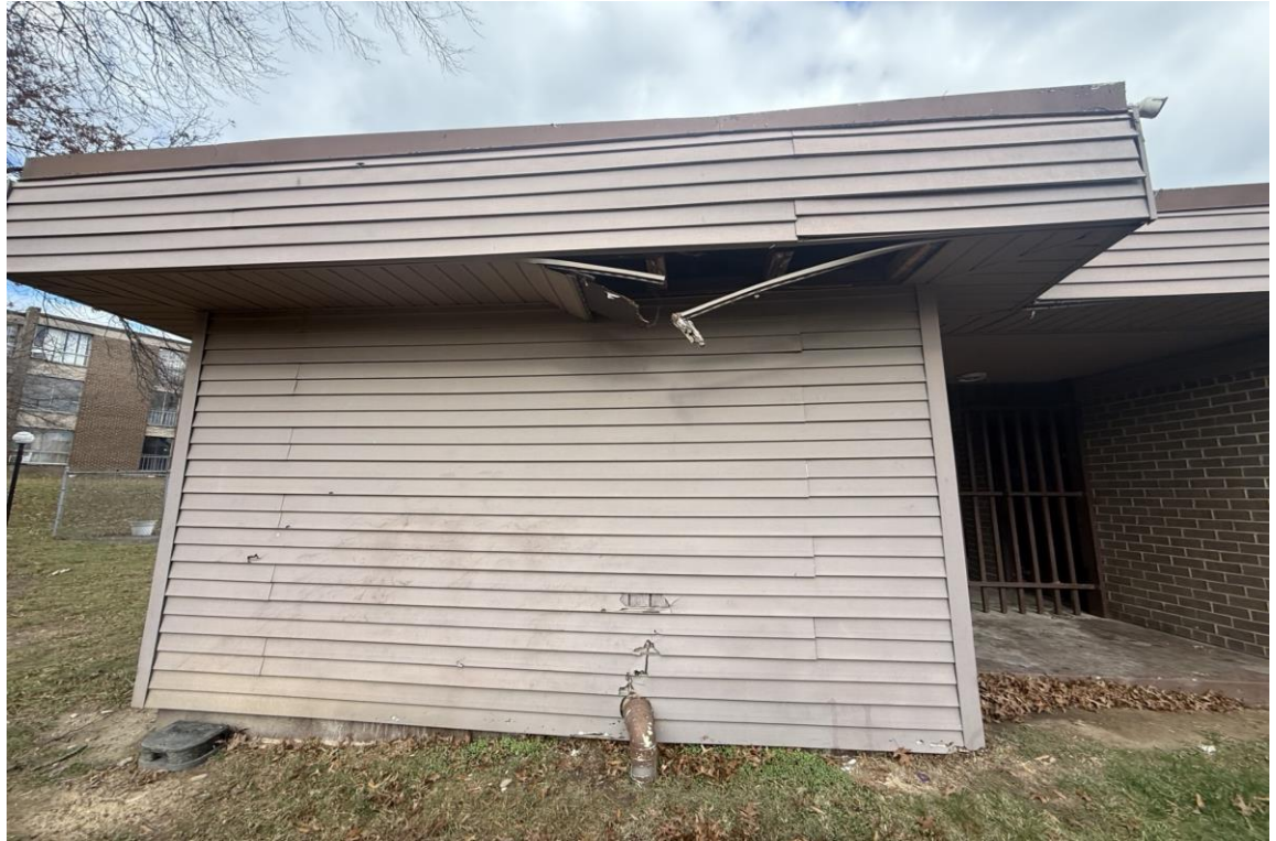
Damaged siding/roof at the façade of the front office 7961 Riggs Rd.
