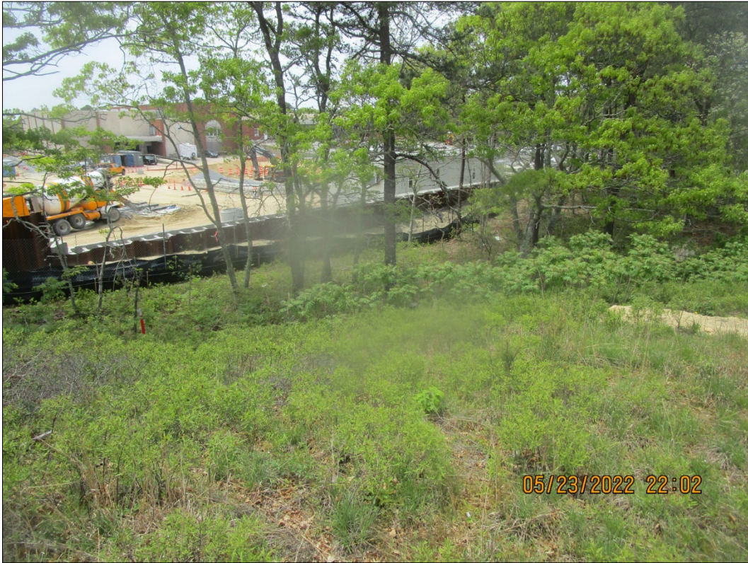
Figure 2. Steep slope in zone of low archaeological sensitivity on Northwest 115kv Cable Duct Bank Route.
