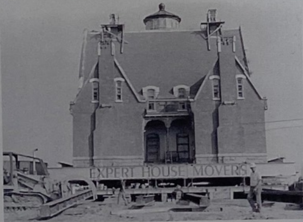
On the first day of the actual move this is what the spectators in the observation tent saw, the building inching forward. Expert House Movers spent most of the summer preparing the light for its very special journey. The actual move was accomplished in about five days, with time out for repositioning the steel tracks for each leg.
